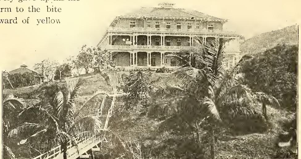
ADMINISTRATION BUILDING, HOUSING THE SANITARY DEPARTMENT
